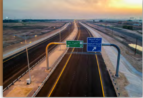
Roads/Bridges and Infrastructure Construction
