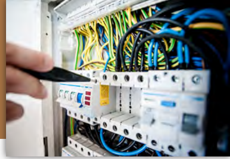
Electrical Engineering Construction
